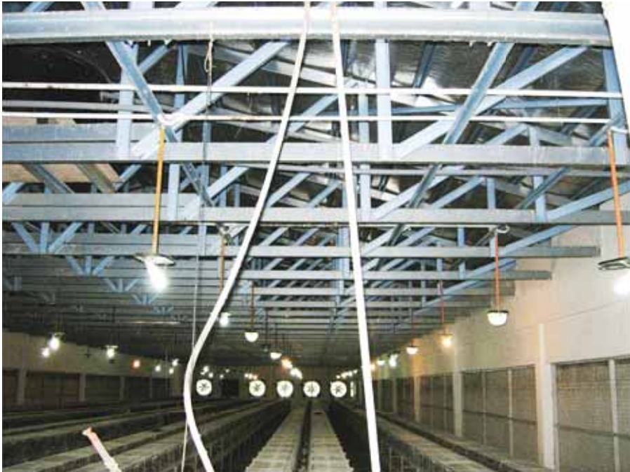
Figure 1. Roof without ceiling
